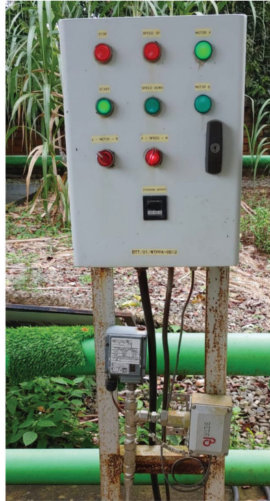
Gambar 4. Pressure Controller
